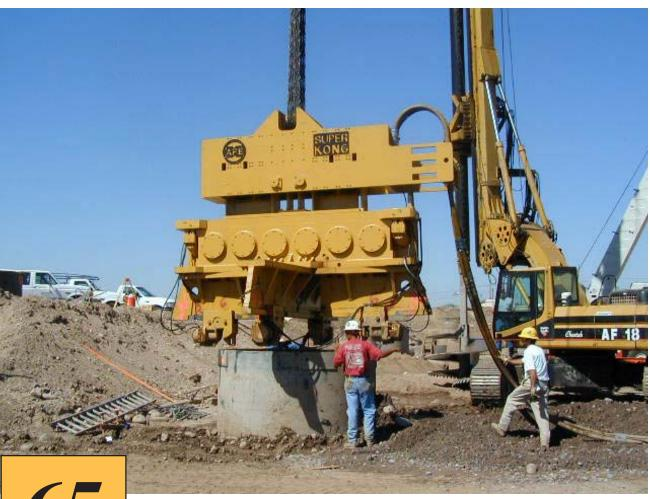
The Model 600 (shown above) is being used as a single unit to drive casings in Arizona. The contractor is Agra Foundations. The 600 vibro is the only vibro that has successfully broken through the rock and cobble layers in Phoenix.
