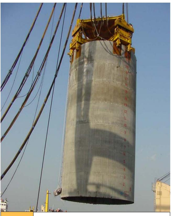
A 40 foot diameter concrete pile weighing over 1.3 million pounds is hoisted using the APE Model 400 Quad. The suppressors are stretched nearly to the limit for over four hours as the pile is transported down river while hanging in the eight jaws of the vibro.
