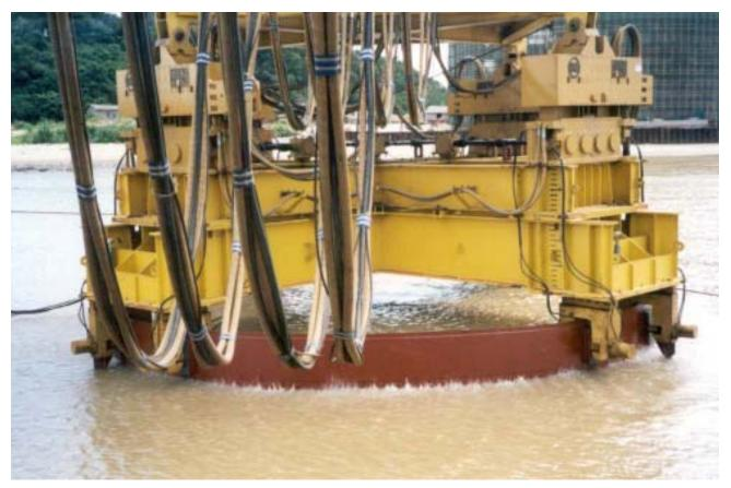
APE Model 400 Quad installs 44 foot diameter caissons in Pearl River in southern China. Piles are over 100 feet long. Soil conditions are up to 50 blow count sands and clay.
