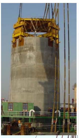
Start to finish driving of the 40 foot diameter concrete pile took under one minute. The pile is 10 inches thick and had more that 50 sensors cast inside it. Total length of the pile was 68 feet.
