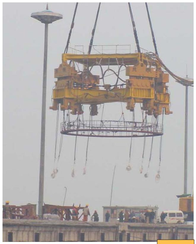
APE Quad 400 shown with all sensor wires hanging from the system as it is about to be placed on the first concrete pile.
