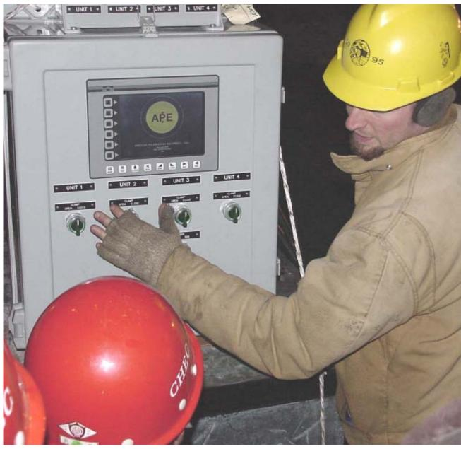
Jimmy Dizard, from Controlled Power, Bellingham, Washington, shows the Chinese pile drivers how the APE monitoring system works. The system controls all four power units at the same time and can display all functions including clamp pressure, drive pressure, engine rpm, vibrator speed and also allows for independent control of each power unit.
