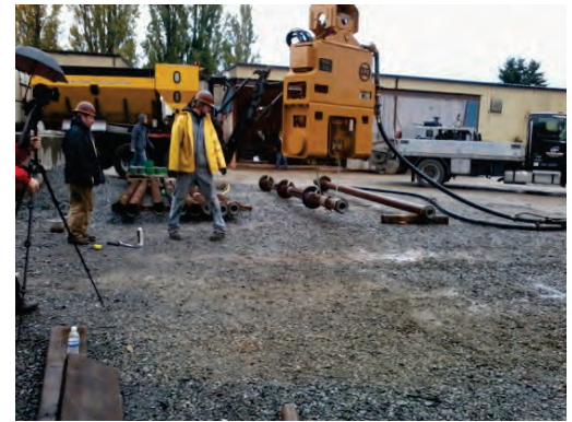
Photo B-2. Picking bottom pile section, Pile 3.
