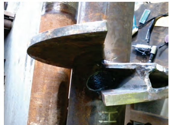
Photo B-3. Pile 4 grout hole.
