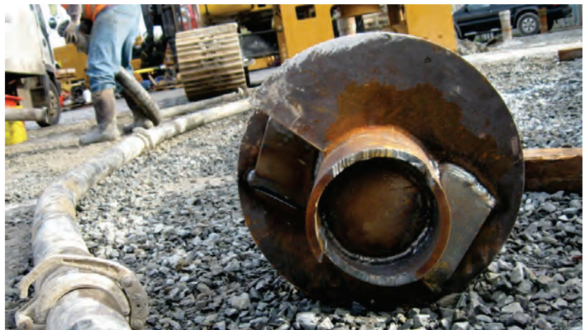
Photo B-4. Pile 5 grout holes.
