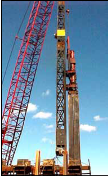
D62-42 in a stand-off driving Kingpile.
