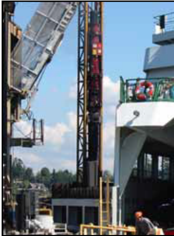
D30-42 Finishing Dolphin Piles.
