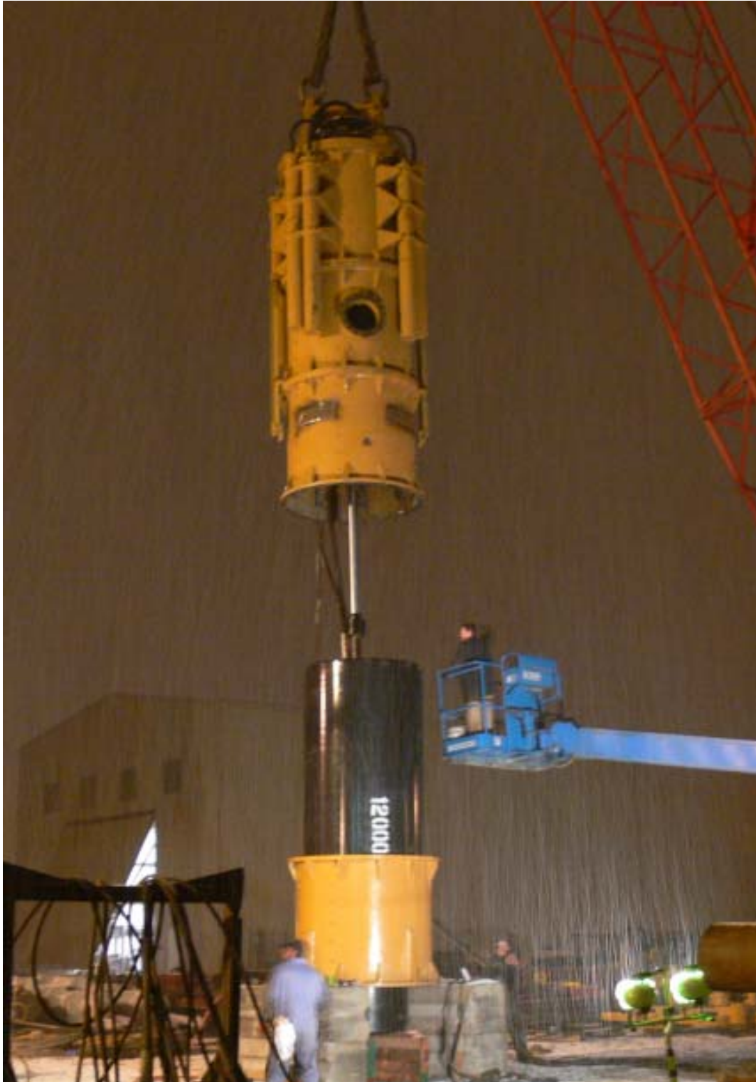
Figure 2-A. Lifting Main Cage & Cylinder onto Bottom Cage
